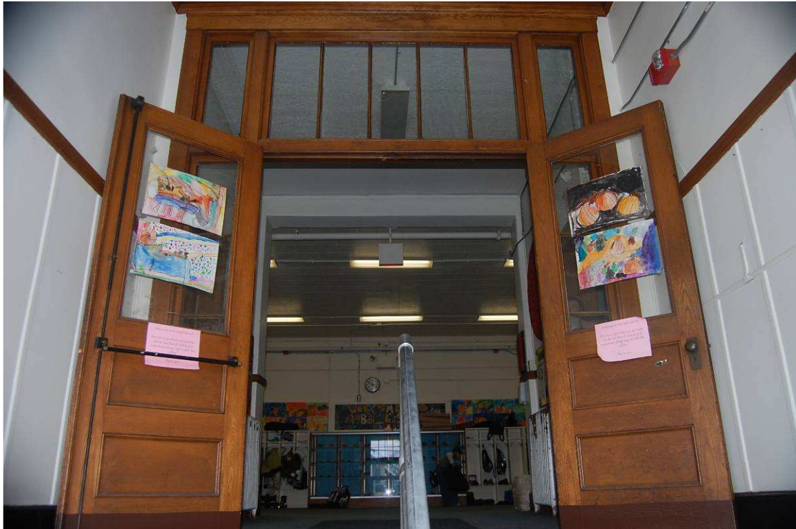
Photo #4 Description: Front vestibule, looking toward 1 st floor hallway Direction: W
