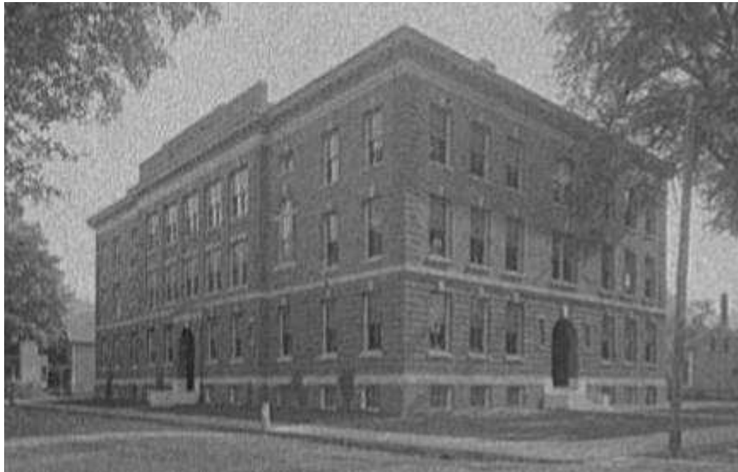
Nashua High School, photographed ca. 1905 shortly after it was completed. Collection of Library of Congress
