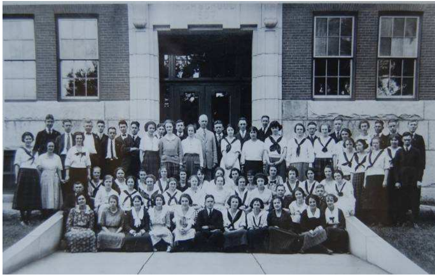
An early class photo at the front entrance to the High School (Kimball School). Note the entablature says "High School / 1907;" this was later changed to "Rundlett Junior High," and even later, "Kimball." Collection of the New Hampshire Historical Society.
