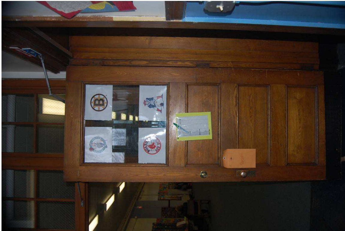
Photo #8 Description: Typical classroom door Direction: S
