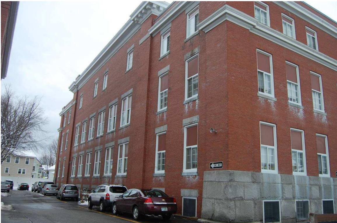
Photo #3 Description: Rear (west) elevation Direction: NE
