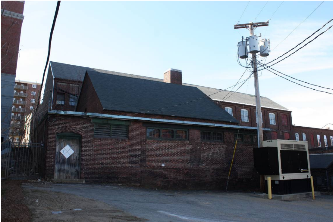
Photo # __6__ Description: Rear (east) elevation of Ford & Kimball foundry with 43-45 S. Main behind Digital file name: CON0291_6 Direction: west
