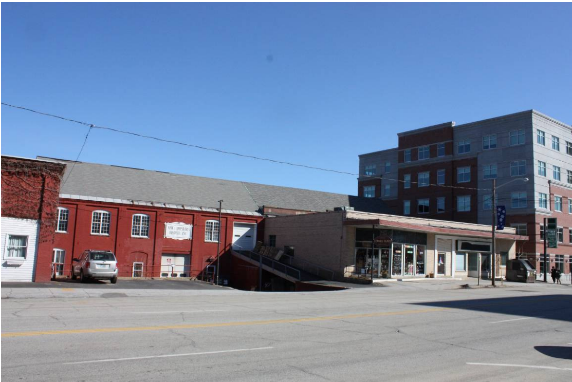
Photo # 5 Description: View from across street, 43 S. Main to left, Smile Building to right Digital file name: CON0291_5 Direction: E-SE
