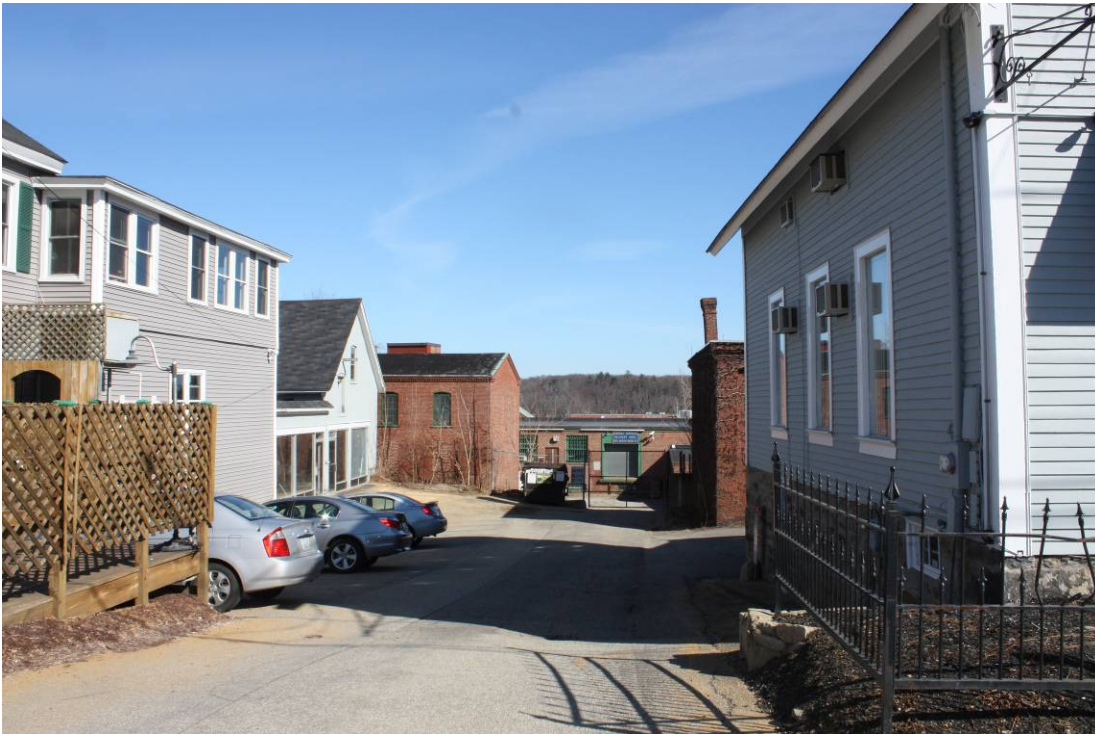
Photo # 12 Description: historic access from Ford & Kimball Office and S. Main to foundry Digital file name: CON0289_12 Direction: east
