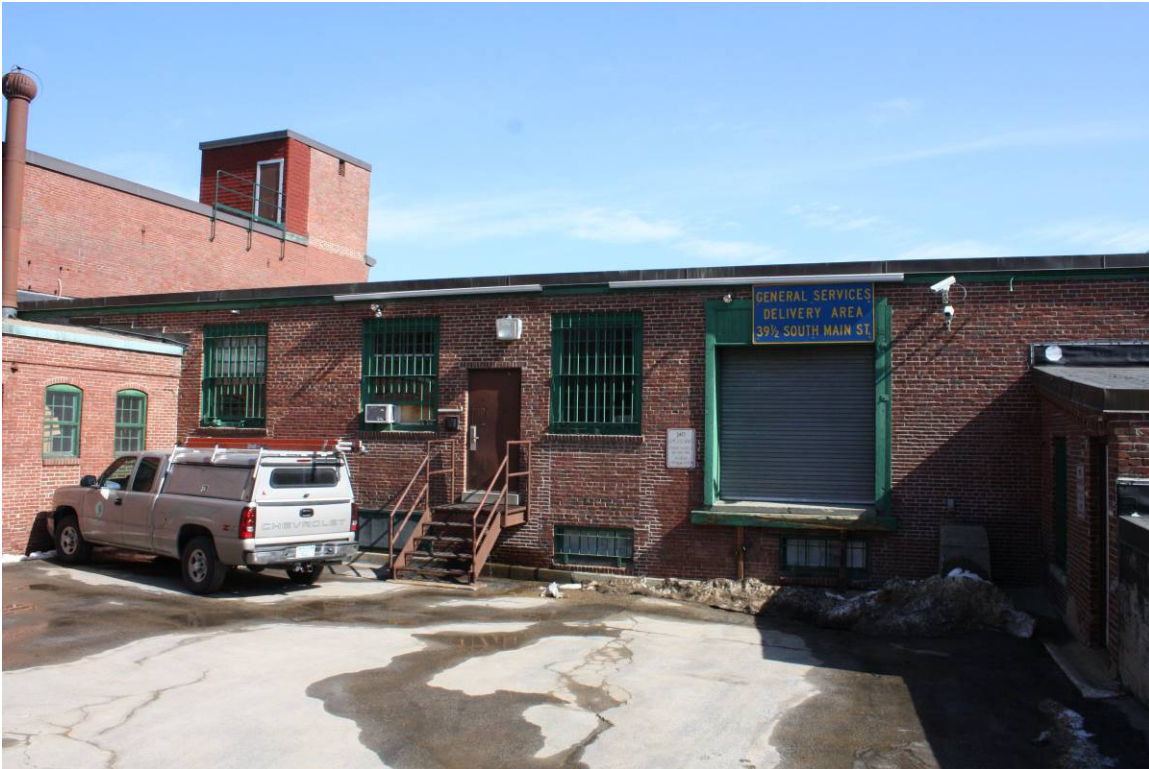
Photo # 6 Description: north end of foundry building, west elevation Digital file name: CON0289_6 Direction: east
