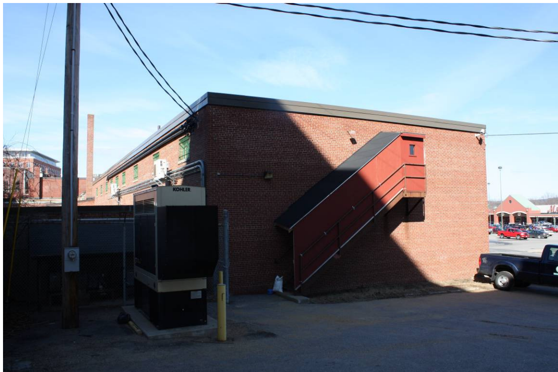
Photo # __9__ Description: Former Foundry, south elevation Digital file name: CON0289_9 Direction: north
