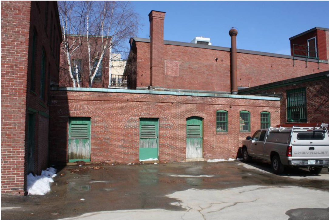
Photo # __4__ Description: Shed/Brass foundry, south elevation Digital file name: CON0289_4 Direction: north
