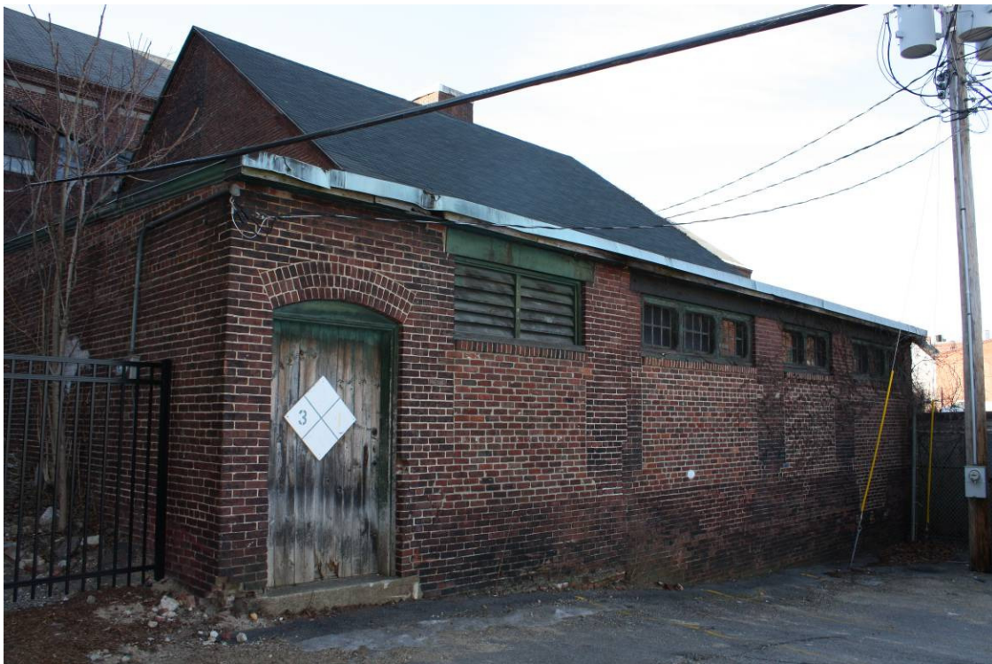
Photo # __5__ Description: Former machine shop, south and east elevations Digital file name: CON0289_5 Direction: NW
