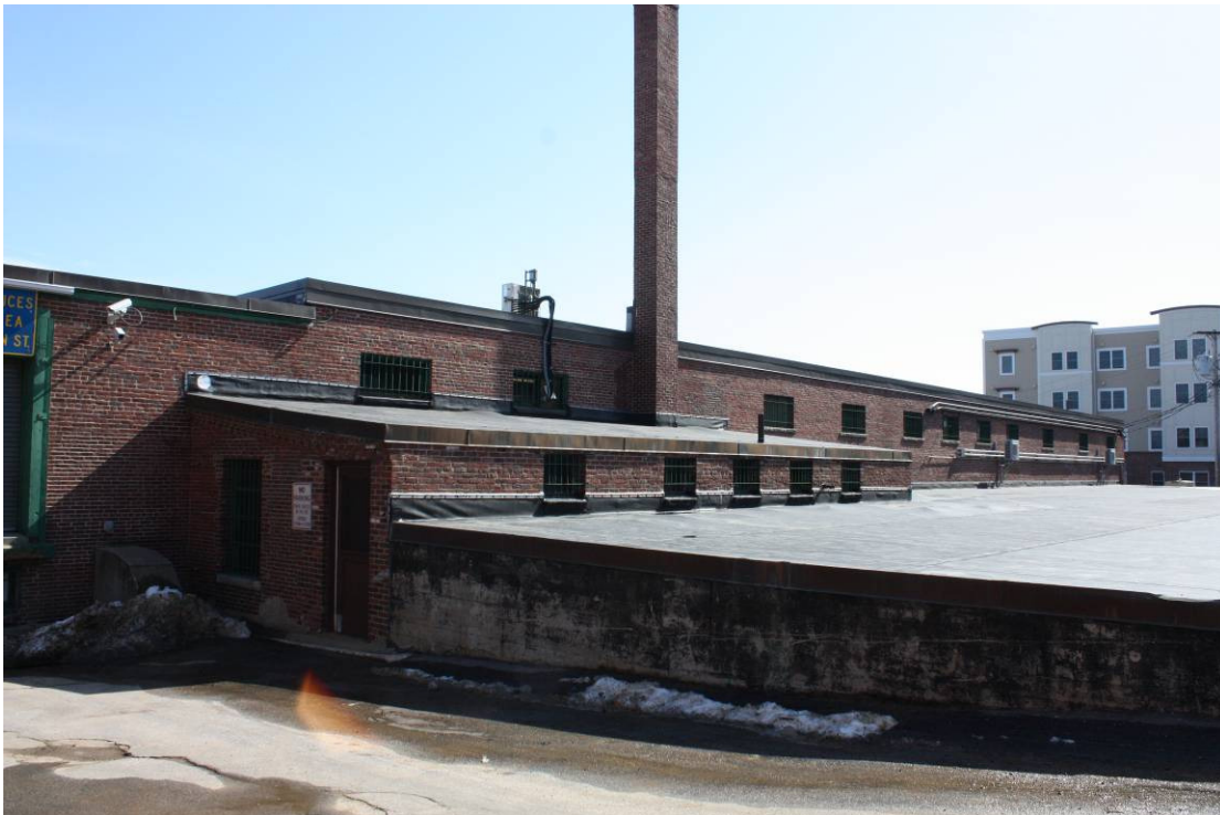
Photo # 7 Description: West elevation of foundry with 1950 addition visible in front right Digital file name: CON0289_7 Direction: SE
