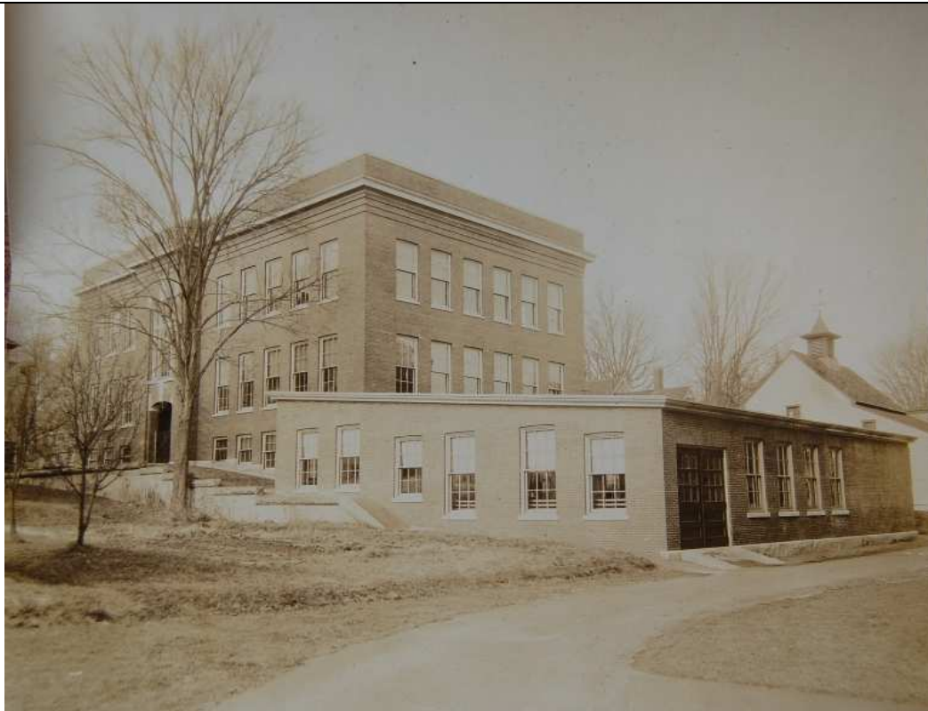
A photograph of the Morrill building, ca. 1927, showing the one-story 1923 addition of a machine shop. The barn at far right is 59 ½ Warren Street, converted to a dwelling by the district ca. 1928. Collection of the New Hampshire Historical Society.
