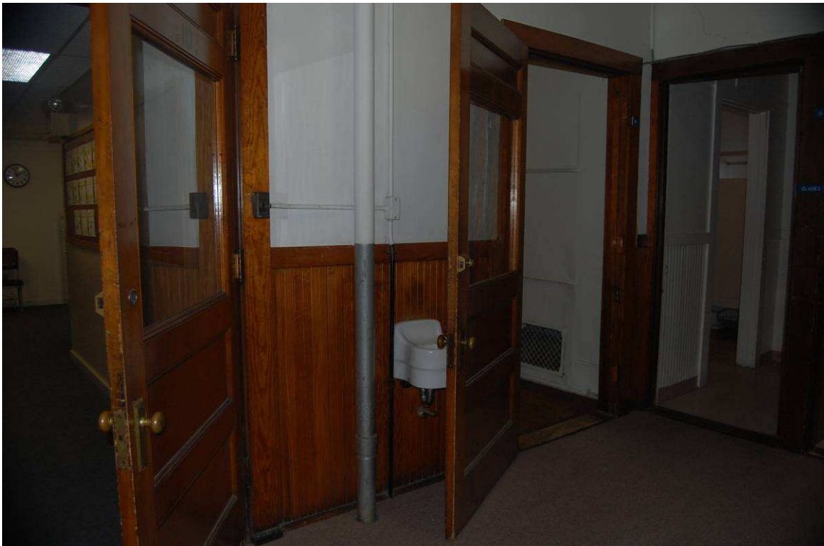
Photo #7 Description: Second floor hall at the top of the stairs in the 1929 addition Direction: SE
