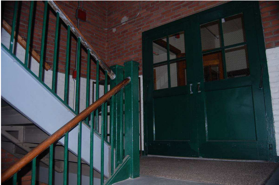
Photo #6 Description: 1929 staircase and interior doors (at north entrance) Direction: SE
