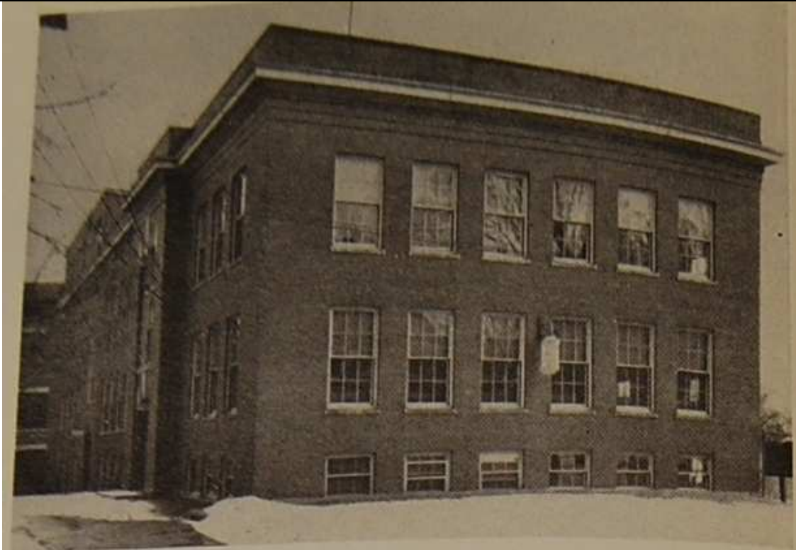
The north and west elevations of the Morrill building as seen in the 1950 Annual Report. Collection of the Concord Public Library.
