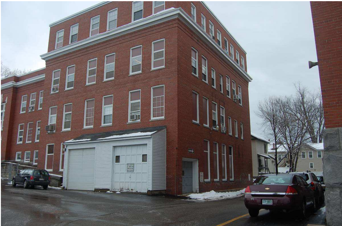
Photo #3 Description: Rear of building, showing 1923 (ground floor) and 1929 (upper three levels) additions Direction: NW
