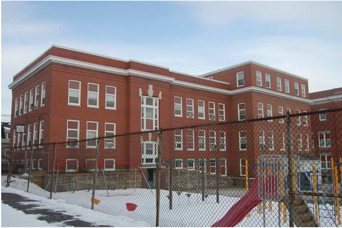
Photo #2 Description: South & west elevations Direction: NE
